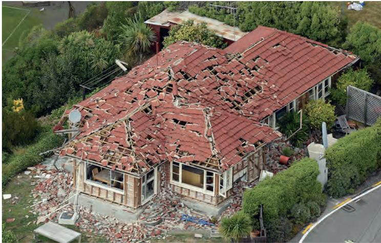
Fig. 1.3 severe damage to a single family house in Light-Weight Timber Construction with non-bearing masonry between the frames and 'heavy' roofing [32]
