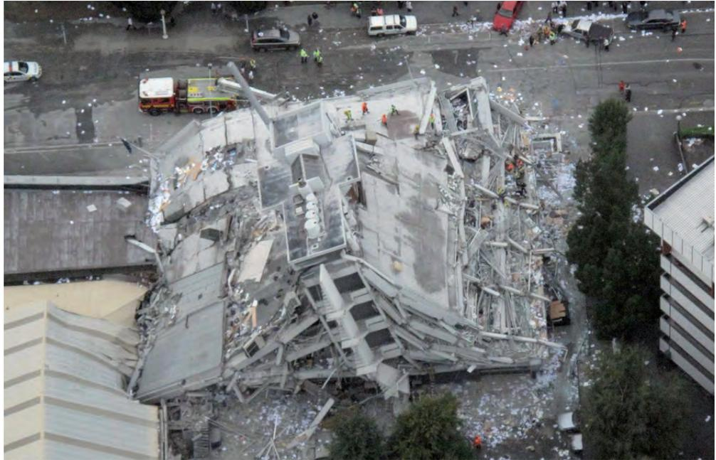
Fig. 1.1 total collapse of a r/c skeleton structure [32]
