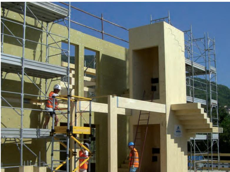
Fig. 1.6 assembly of a staircase with a central lift core shaft [34]
